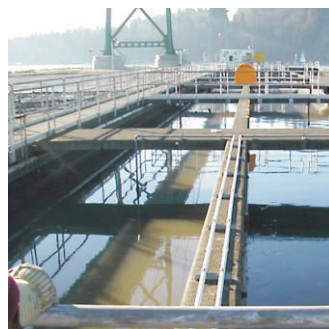
Lions Gate Waste Water Treatment Plant
