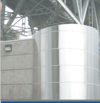
Granville Pump Station
