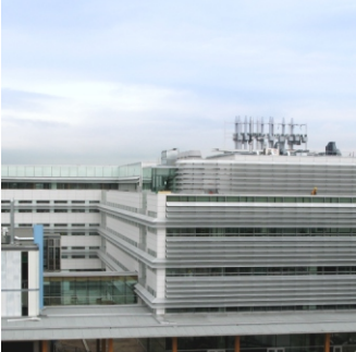
UBC Earth Science Building
